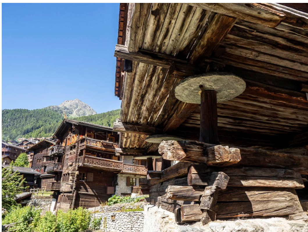
15 Traditional Valais architecture – stone slabs keep mice away from grain stores
